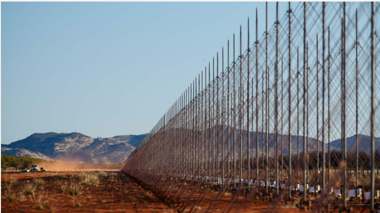
Jindalee Operational Radar Network © 2016 BAE Systems.
